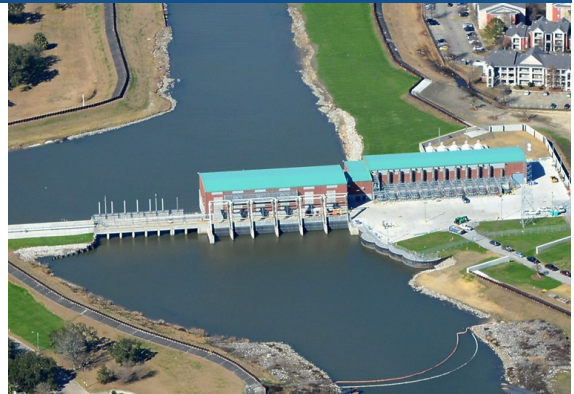
London Avenue Canal PCCP
