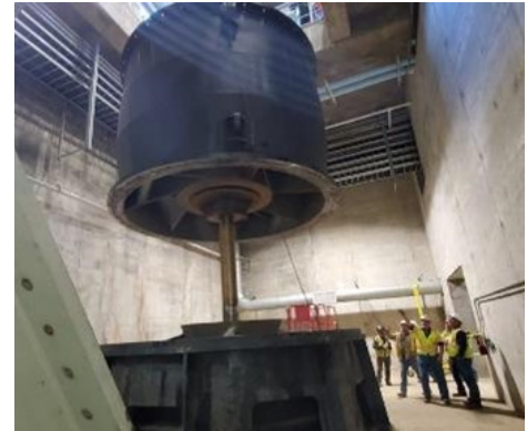
Diffuser section removal
